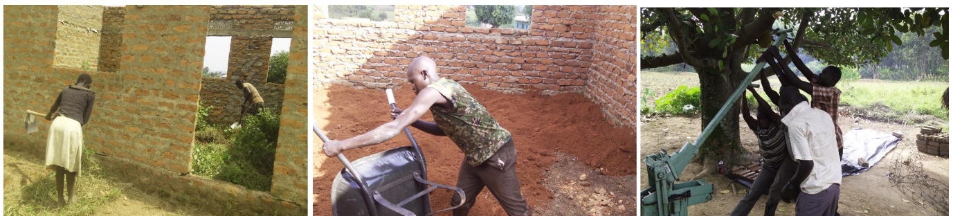
.....Some of the works that took place at the site.....
